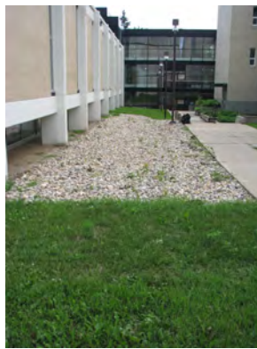
Figure 7. Gravel bed, SW side of the original Health Studies Building.
