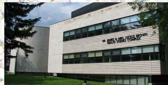
Figure 4. Tyndall Stone walls, Health Studies Complex.
