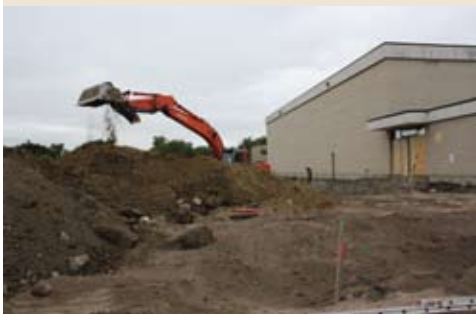
Construction began in August on the Healthy Living Centre.
