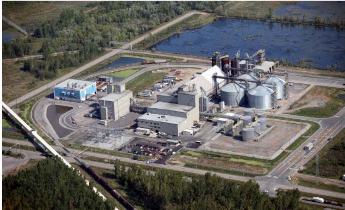
Viterra Soybean / Canola Processing Plant, Becanour, Quebec (1.05 M tonnes/year)
