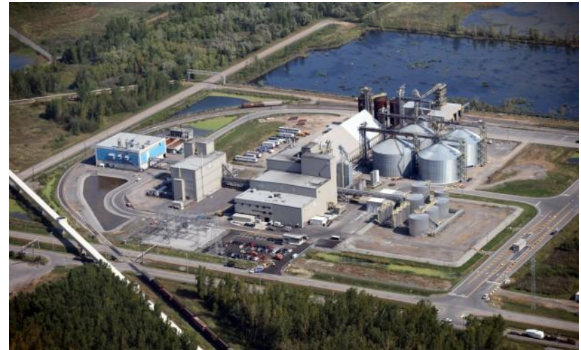
Viterra Soybean Processing Facility Becancour, QC
