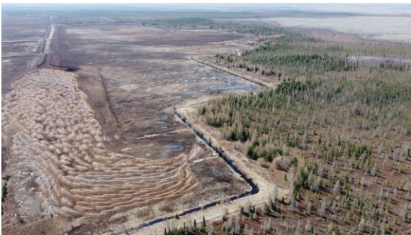
Drone's eye view of the restoration project site near Elma, Manitoba.
